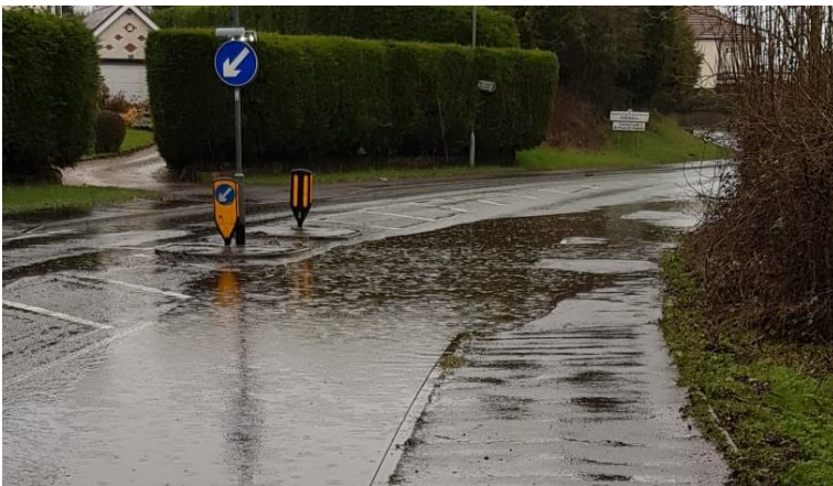
Flooding on Lane Green Road
