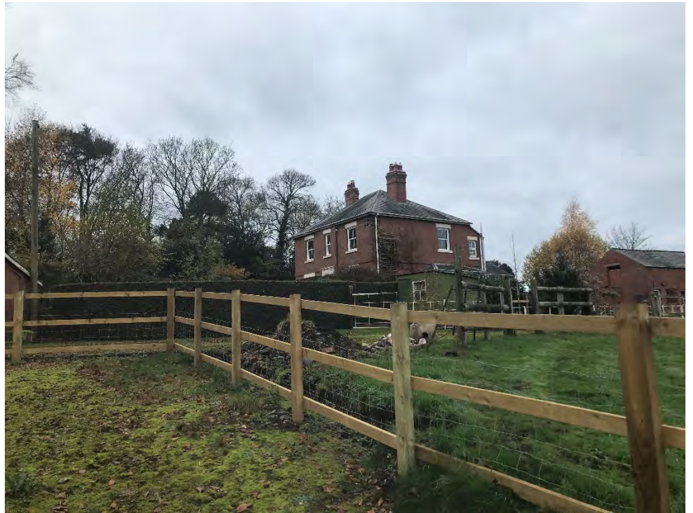
Plate 8 Southeast elevation of the early 20 th century un-listed Newhouse Farm. Image taken from the western boundary of the subject site.
