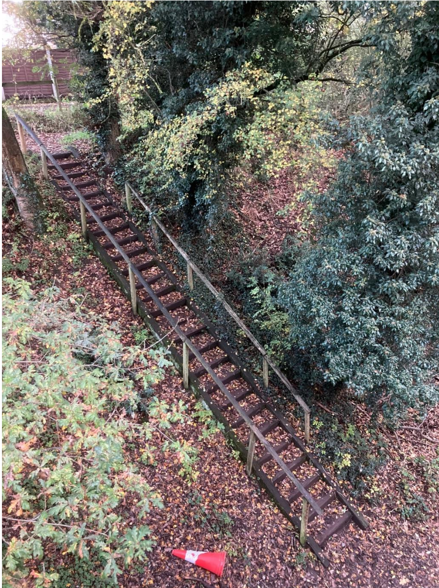
Steps down to railway walk at north of proposed site 582
