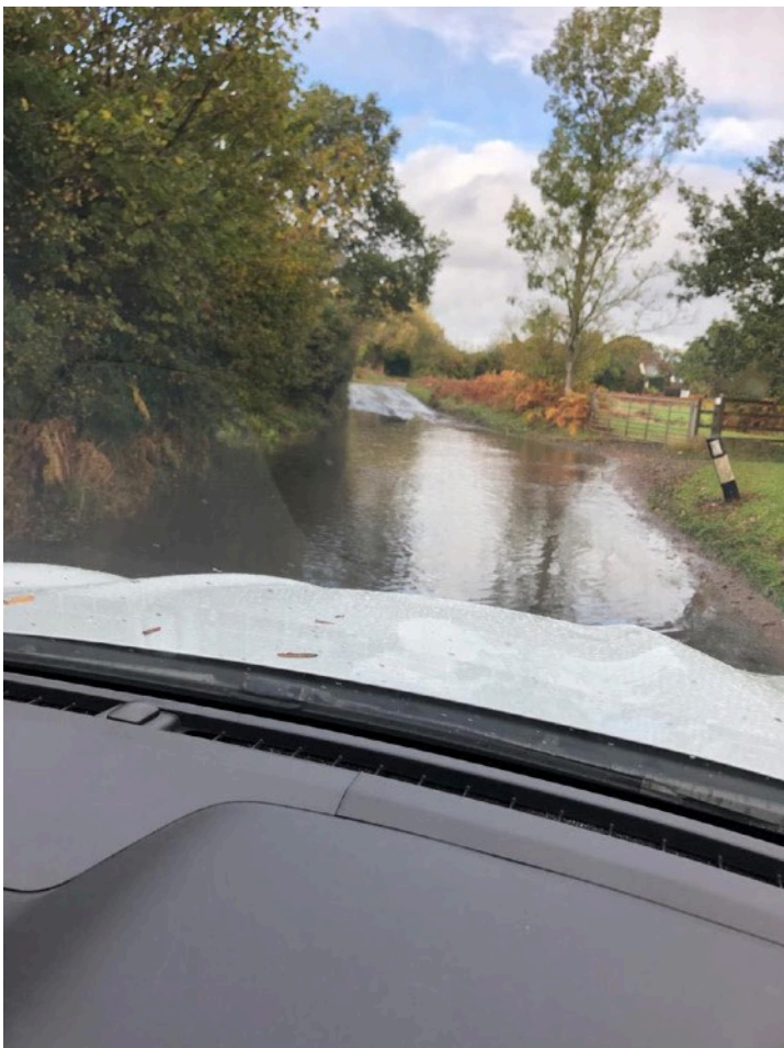
Radford Lane, Lower Penn. The same bend as above pictured travelling away from Langley Road. The flooding pictured here is typical in this location.
