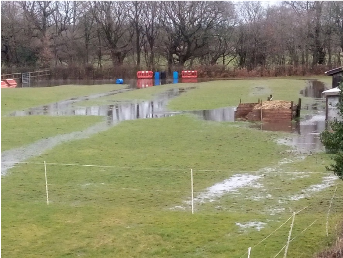
Heavily waterlogged land due to run off from adjacent fields and high water table. Map point E
