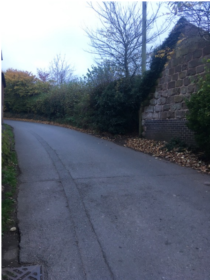
Springhill Lane, Lower Penn. No pavement, with a public footpath the emerges directly onto the carriageway. A tight bend on a narrow road.
