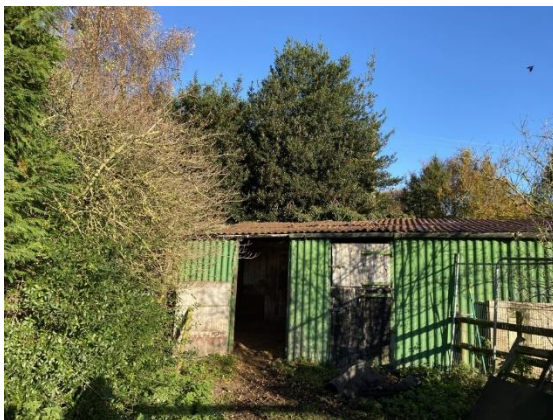
Photograph 5. View of on-site structure, looking north
