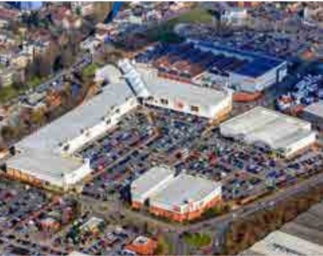
Bentley Bridge Retail Park
