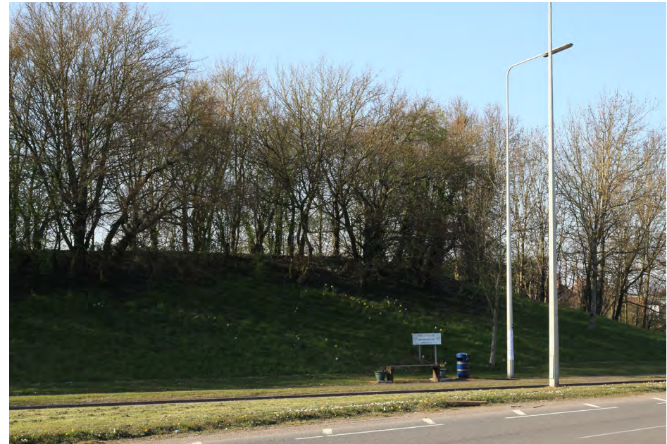
Figure 8: Embankment to Eastern boundary of the site
