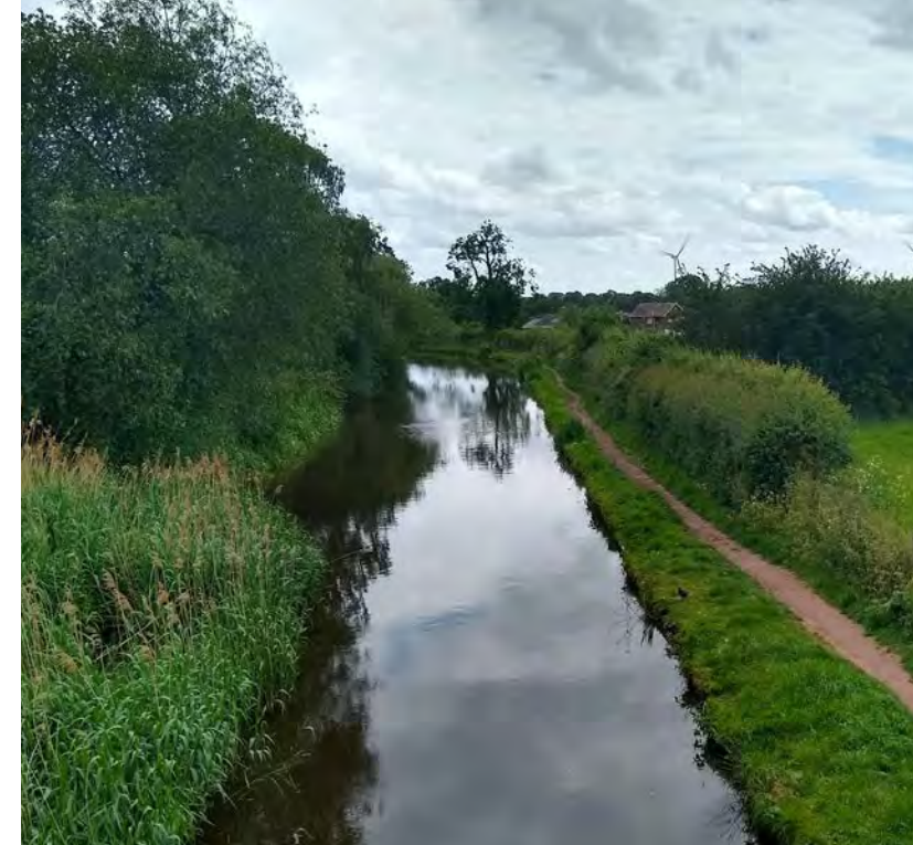
STAFFORDSHIRE AND WORCESTERSHIRE CANAL
