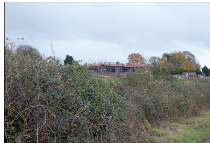
Photograph 1 – Partly Constructed Nursery
