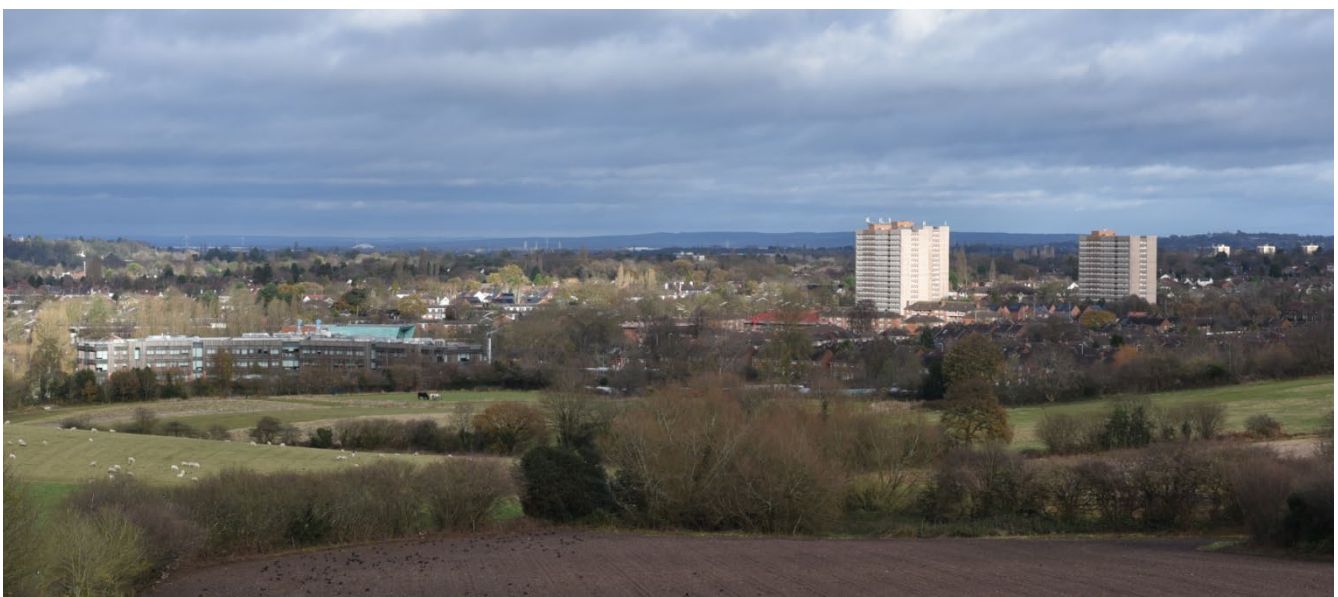
Figure 10 Merry Hill Tower Blocks and Highfields School
