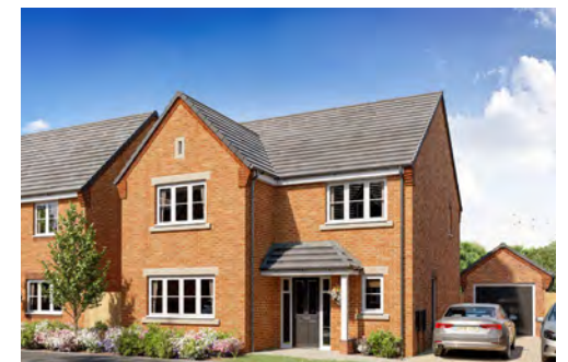
Seven Homes | Mixed Development Homes
