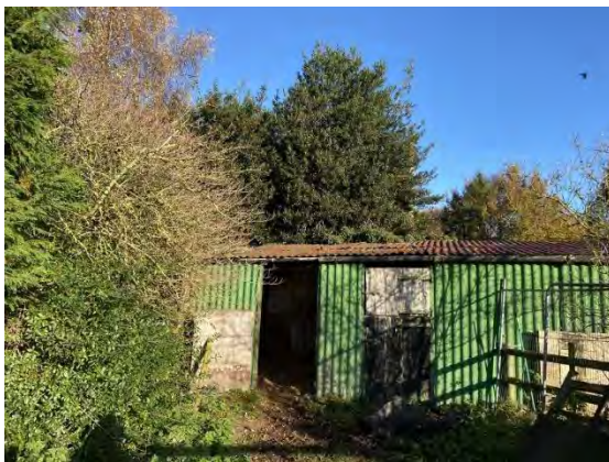
Photograph 5. View of on-site structure, looking north
