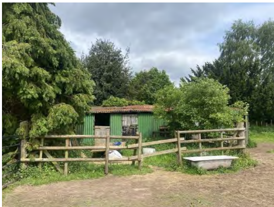
Photograph 5. View of on-site structure, looking north
