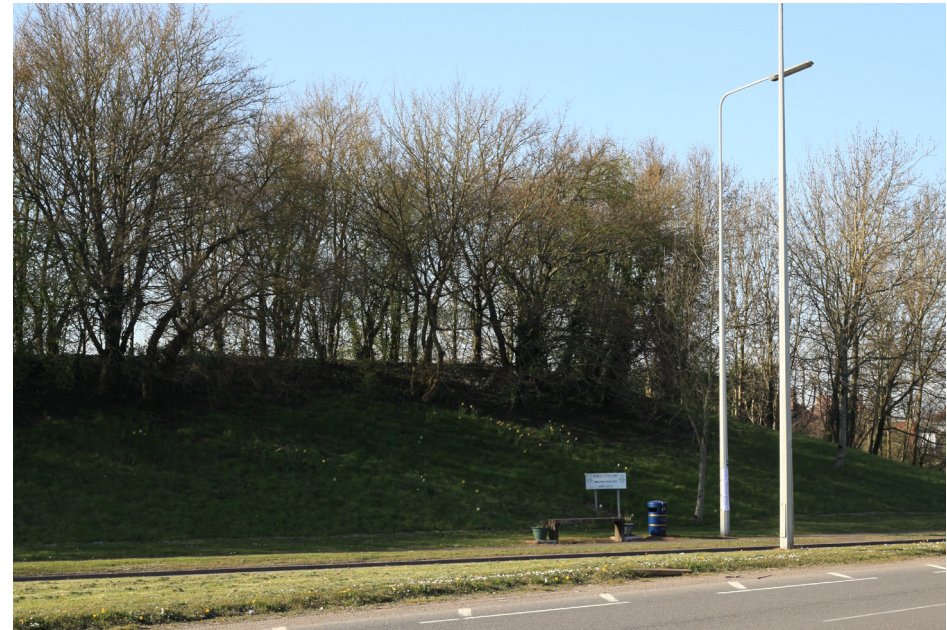
Figure 8: Embankment to Eastern boundary of the site
