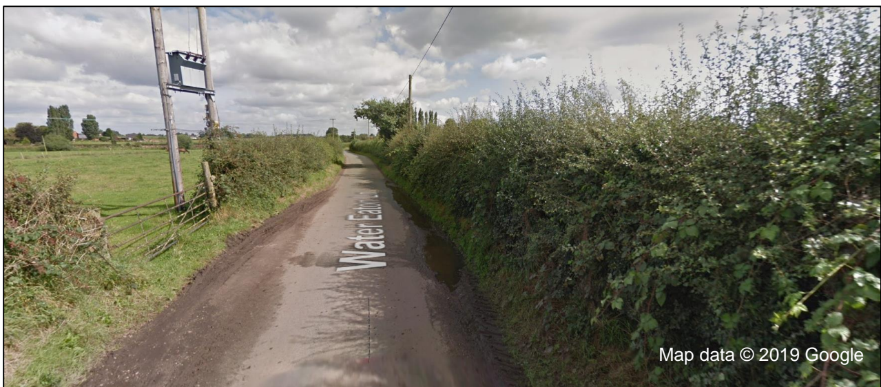
Figure 3-6 - Water Eaton Lane
