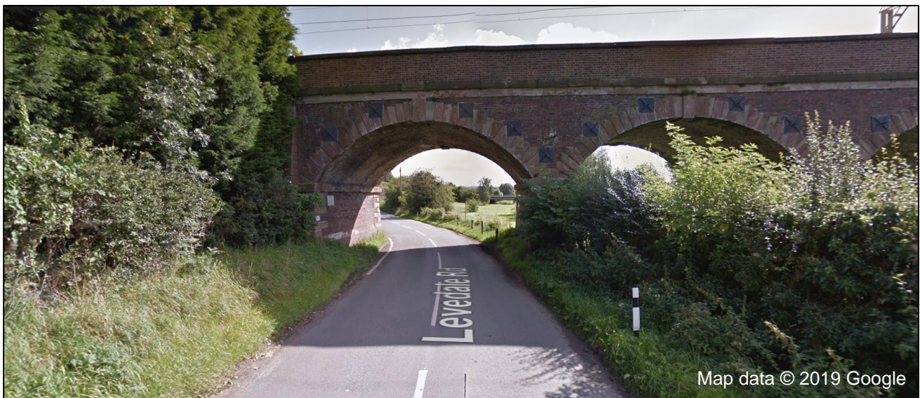
Figure 5-6 - Levedale Road - Tunnel
